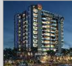
Archi Platinum Sukhadiya Circle
