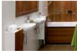
Bathrooms: Washbasins and WCs in different shades; Chrome plated tap fittings; hot & cold water supply
