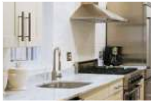
Kitchen: Finished Granite stone platform; stainless sinks; glazed title Dado on wall up to 2 ft over counter
