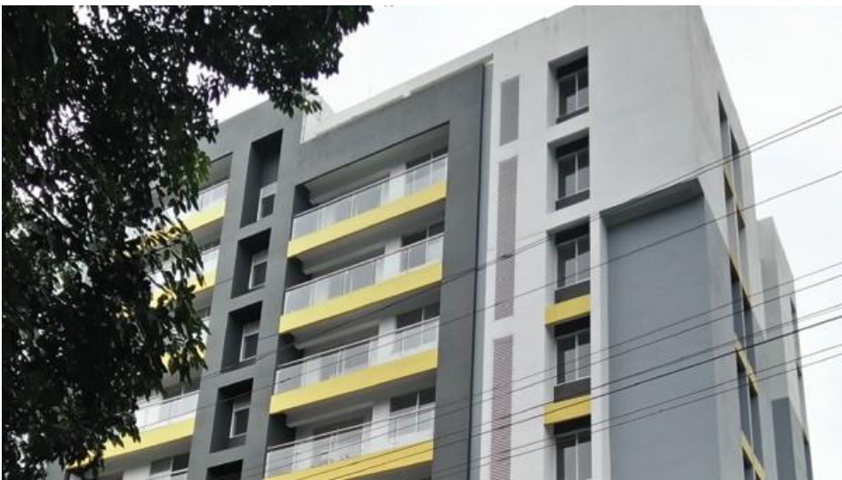
VANILLA GROVE APARTMENTS, KOLENCHERY
