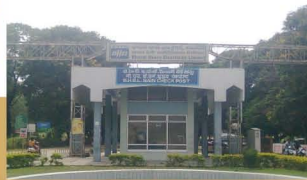
BHEL (Bharat Heavy Electricals Limited)
